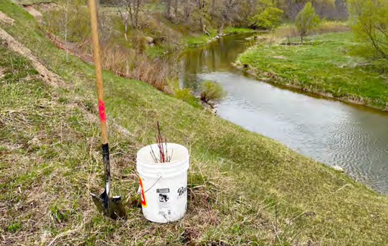
Tree, shrub, and plant roots help stabilize a bank and reduce erosion.
